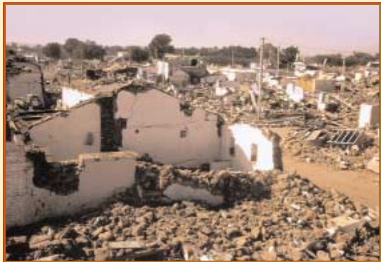
The village of Dhamadka a few days after the 2001 earthquake.
